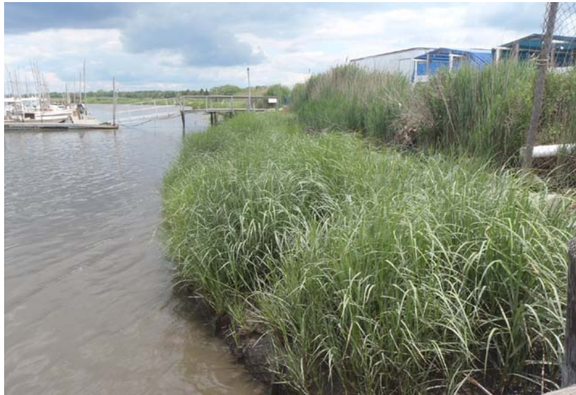
Figure 28. Example of living shoreline constructed of natural fiber logs and mats, oyster shell, and seeded with mussels and vascular plants.
